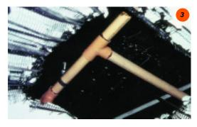
Davidson used pendent heads in all dwelling units, which required a flexible piping material such as BlazeMaster® CPVC pipe that could be installed with only a 2' X 2' opening in the plaster on lath ceilings (Photo 3). In the corridors, the piping was concealed behind one-hour fire rated constructed soffits because of structural steel beams obstructing the path of the sprinkler feed mains (Photos 4 and 5).
