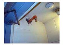
According to Heller, when steel fire sprinkler systems are installed, the inhabitants of an entire floor must be evacuated. Also, messy cutting oil or pipe dope can damage carpeting in the residents' apartments.
