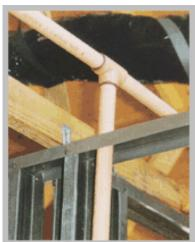
One of the biggest advantages of BlazeMaster® fire sprinkler systems is the ease and speed of installation. Fred Benn noted, "because the CPVC pipe is so light in weight and has some flexibility our installers are able to install the system more quickly compared to other materials and this enables us to stay ahead of the developers' schedule, which translates into cost savings for us and the developer."
