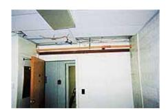
The first residence hall at Wake Forest was retrofitted with a steel fire sprinkler system, which proved to be time and labor intensive. The design of the steel fire sprinkler system required extensive field survey, which could not be performed until students vacated the residence halls for summer recess. And, design and fabrication pushed the installation period perilously close to the date students returned from summer vacation.
